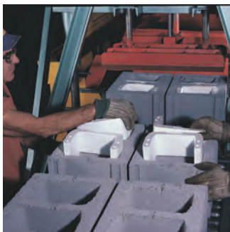
Block plant installed
